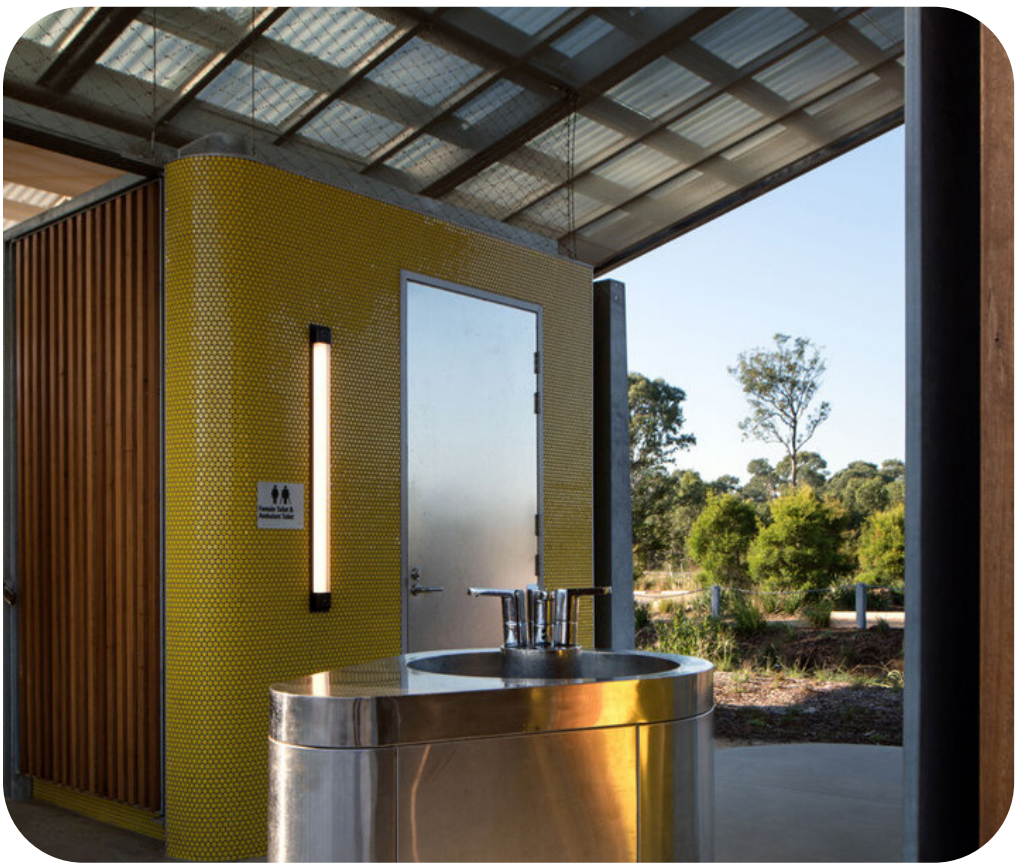
The toilet cubicals can be read as pods with their own internal ceiling whilst retaining the high ceilings and truss structure in the communal areas.
