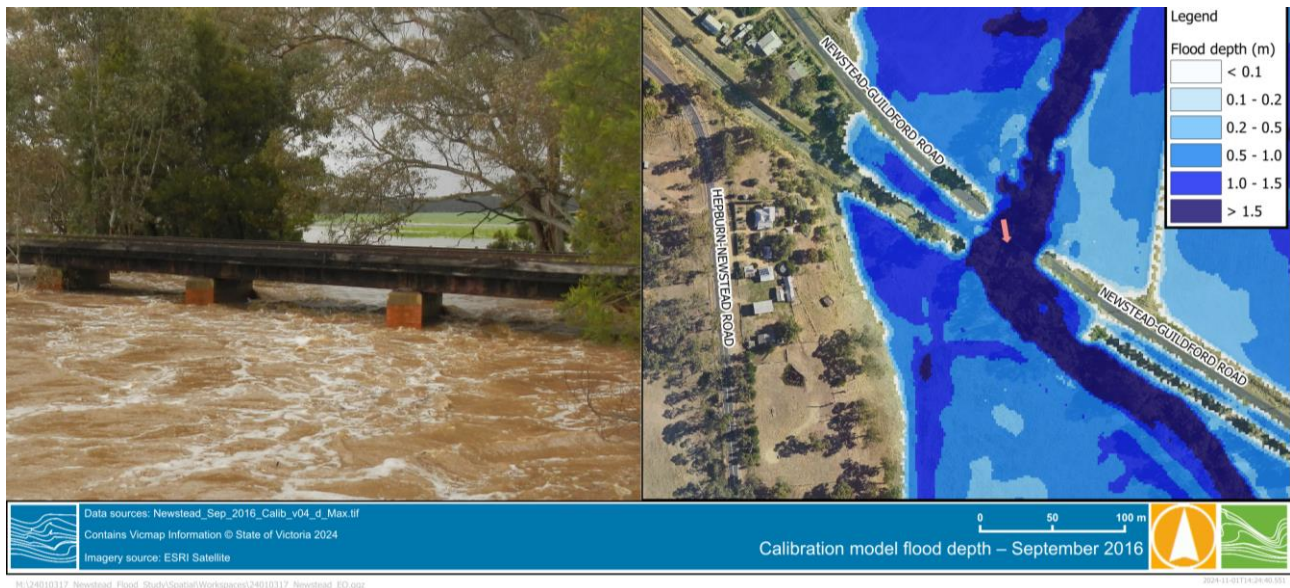
Figure 4-14 Railway bridge over Larni Barramal Yaluk, captured at around 1130 hours on 14 September 2016. Agrees well with modelled peak flood extent and level (modelled level is approximately 0.5 m below bridge soffit).
