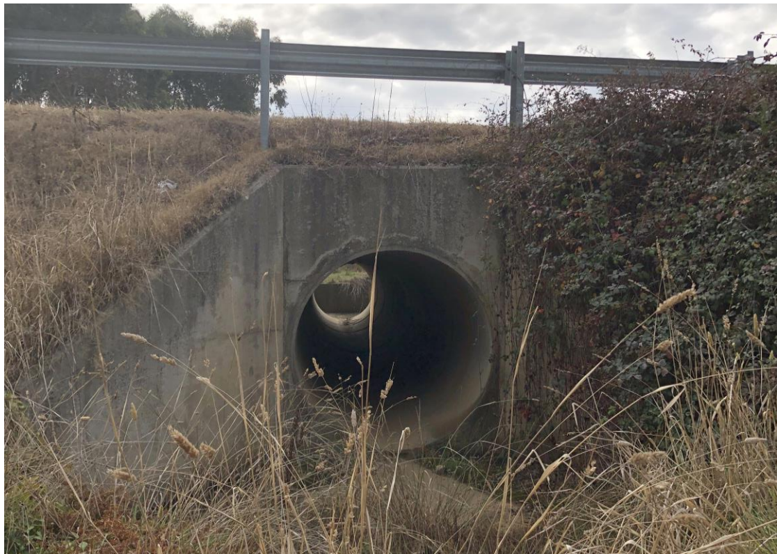
Figure 6-7 Pyrenees Highway culvert at Green Gully
