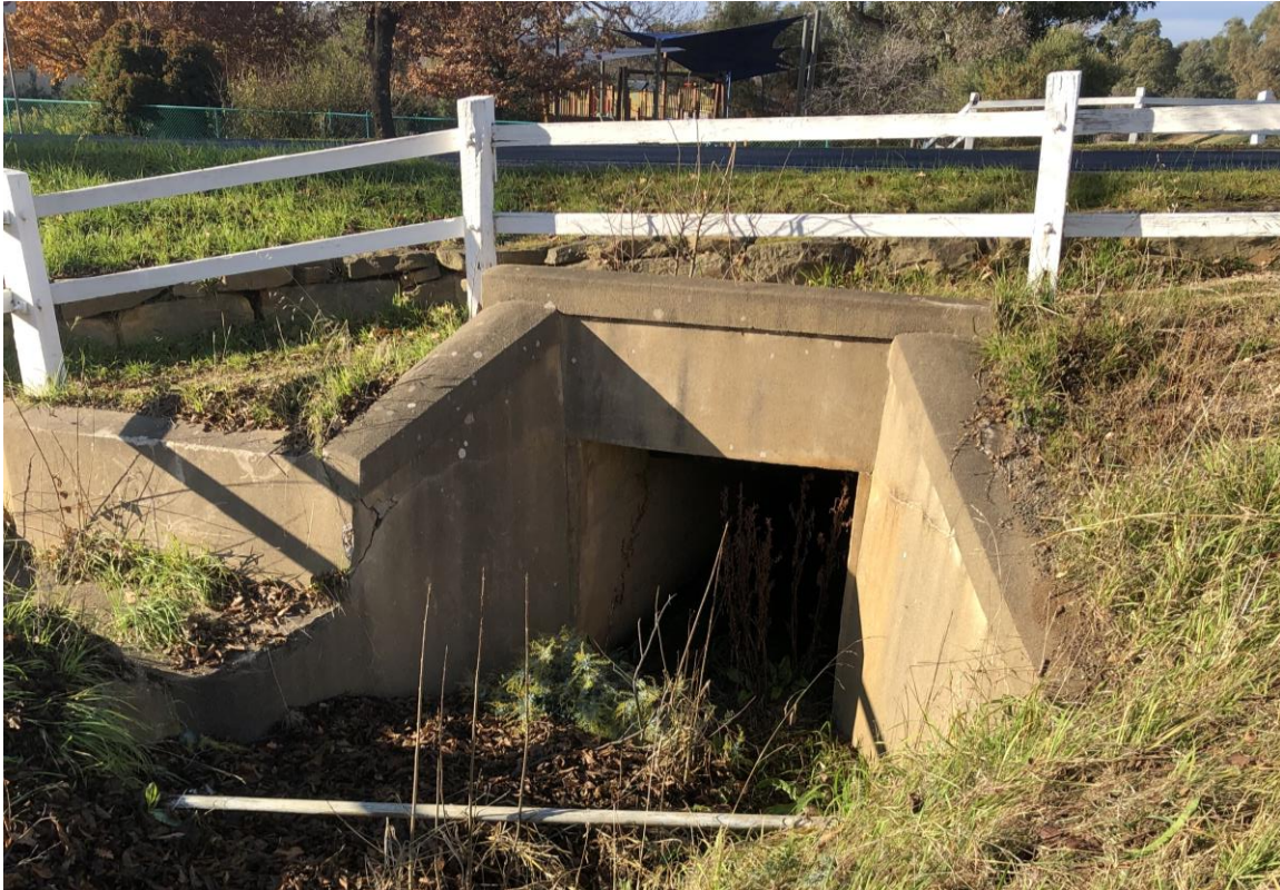
Figure 6-1 Culvert under Pyrenees Highway/Lyons Street directly east of levee
