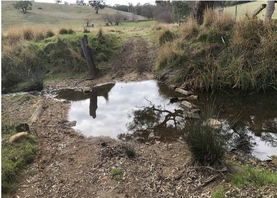
Figure 6-6 Muckleford Creek floodway at Palmerston Street
