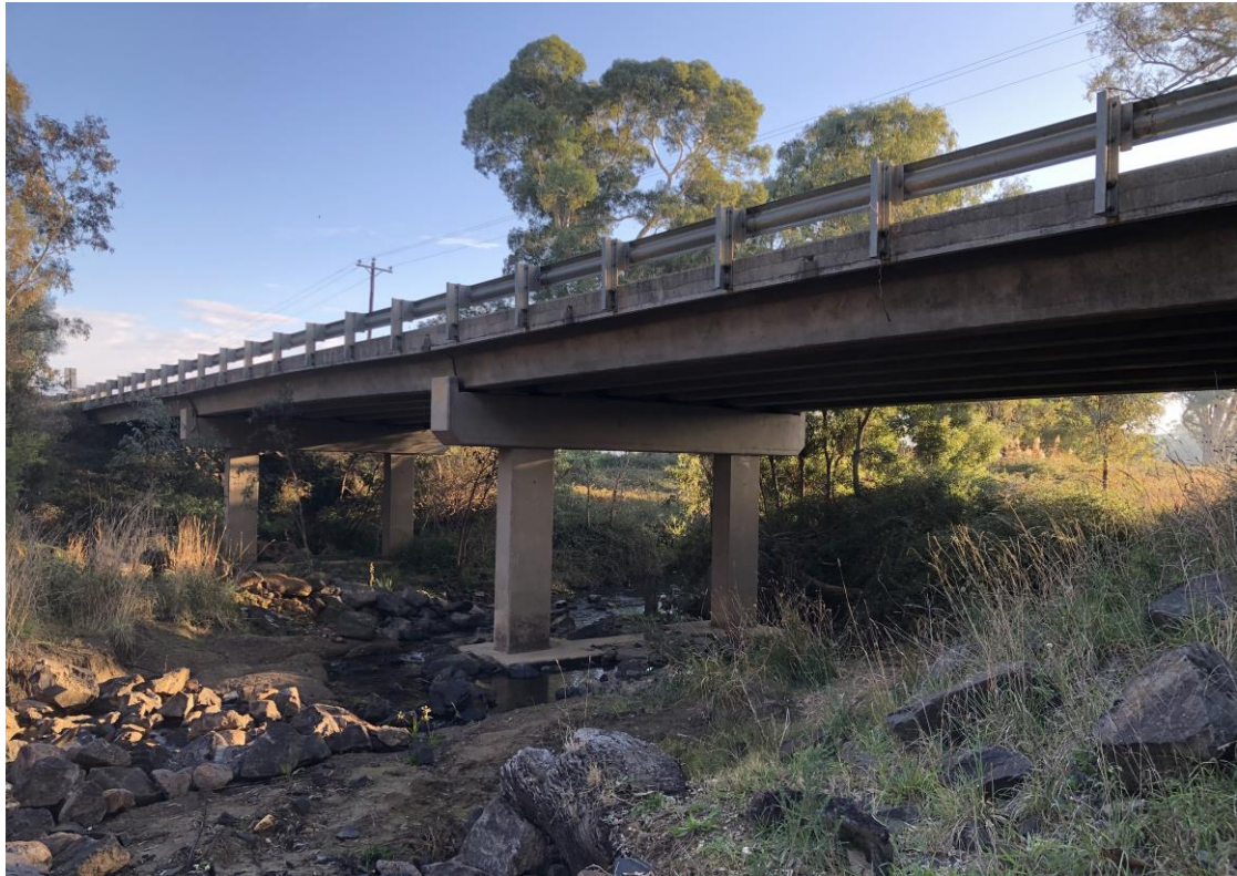
Figure 6-4 Newstead-Guildford Road bridge over Larni Barramal Yaluk
