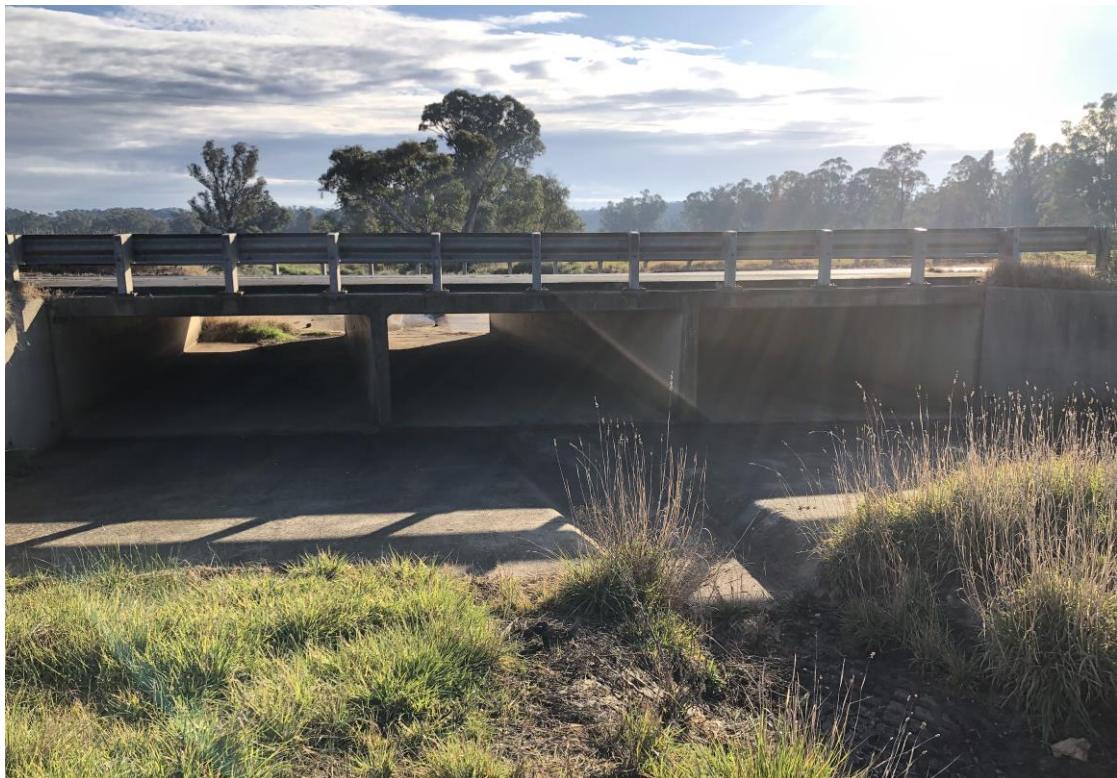
Figure 6-3 Pyrenees Highway culvert at Green Gully Creek
